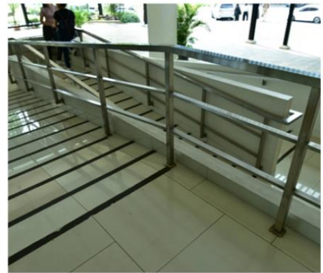
Permanent wheelchair ramp for the disabled
